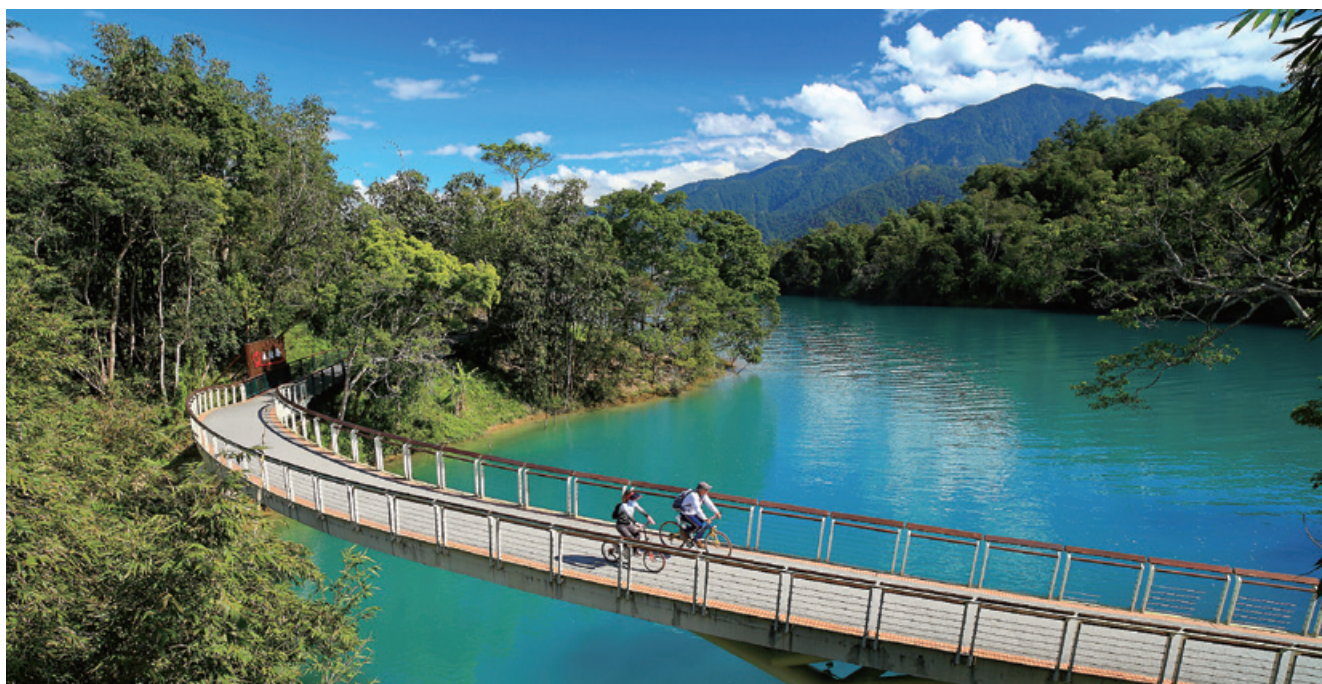
Yongjie Bridge ©TTA
